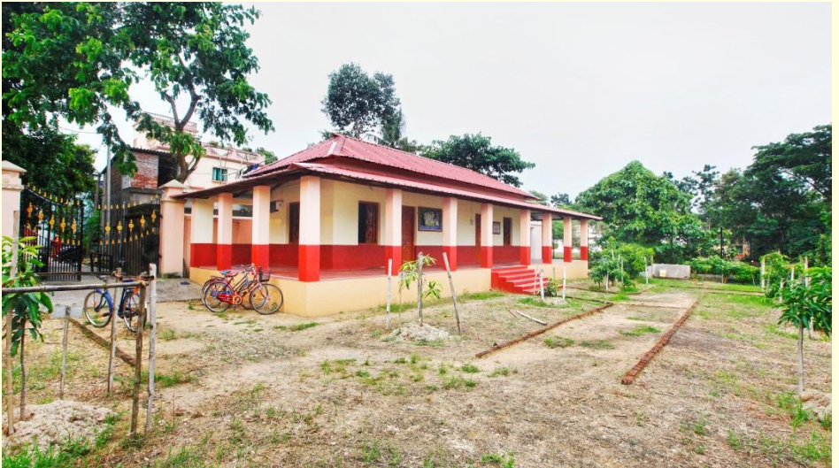
Mango Grove Administrative Building
